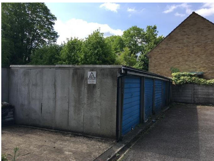
Photo 5: external view of garages, showing single block concrete walls and flat roof.
